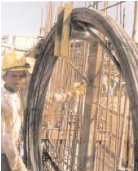
Reeled monostrands being installed during slipforming
