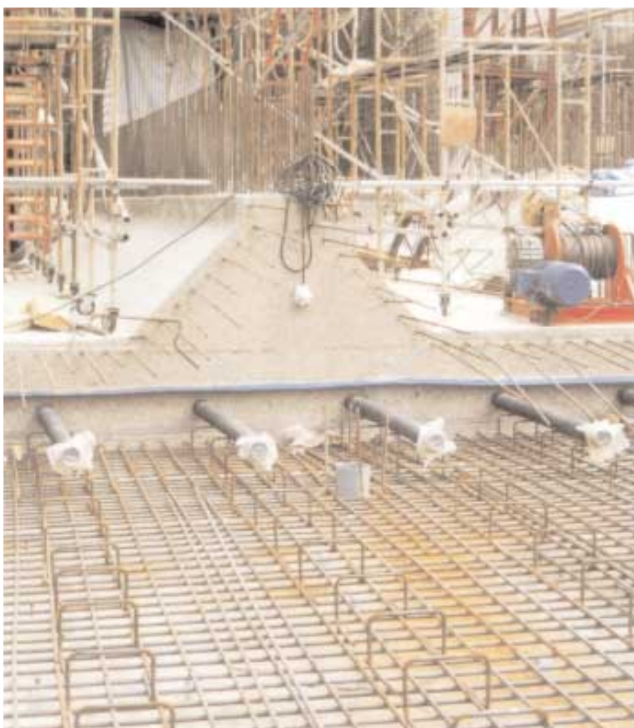
Construction Joint Base Slab
