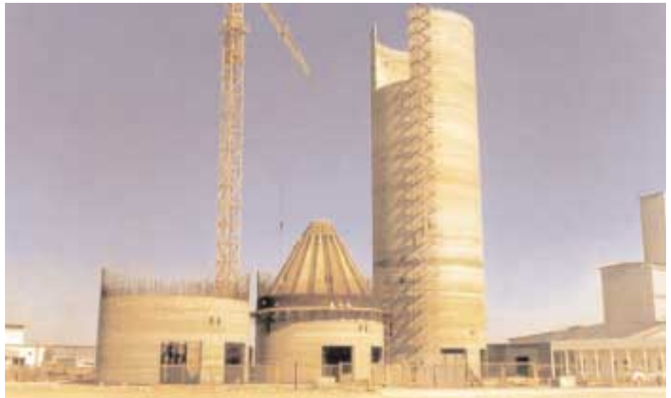
Slipforming in progress on Clinker Silo
